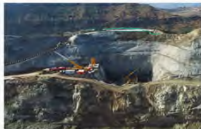
INTAKE & POWER TUNNEL
