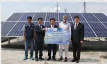
Solar Panel for Kotli School
